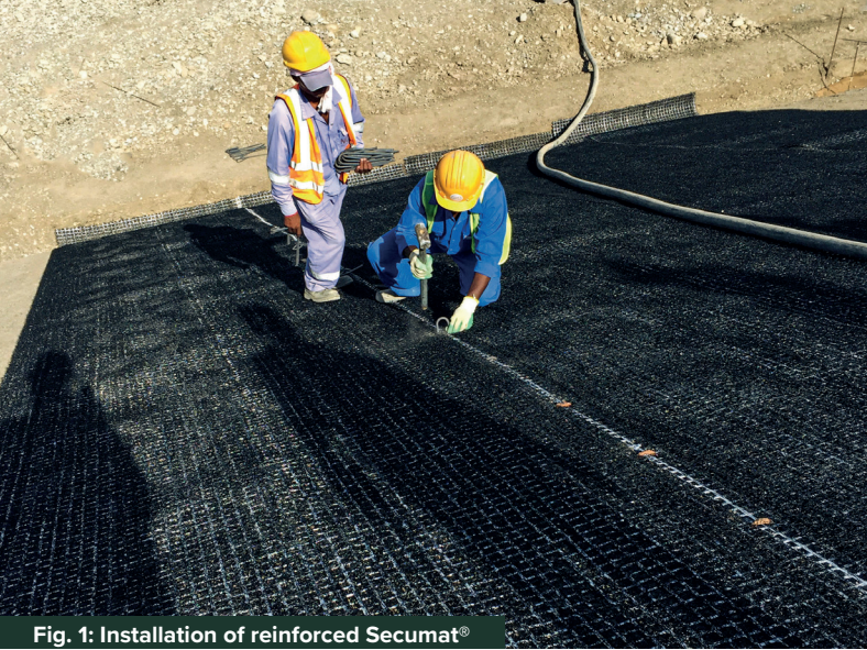
Fig. 1: Installation of reinforced Secumat®
