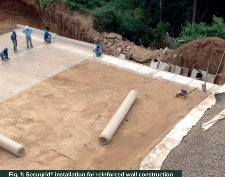
Fig. 1: Secugrid® installation for reinforced wall construction
