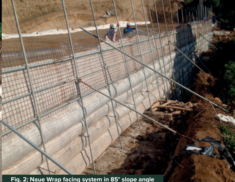
Fig. 2: Naue Wrap facing system in 85° slope angle
