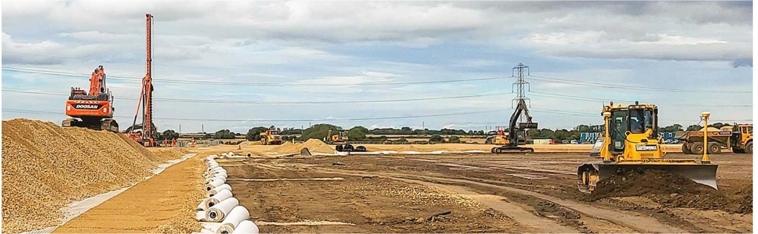
Naue have supplied Combigrid® and Secugrid® products for use in the construction of working platforms, to support piling and crane operations, during construction of a gigafactory which will span 50 hectares of land at the International Advanced Manufacturing Park (IAMP) in the north east of England, on the border between South Tyneside and Sunderland.
