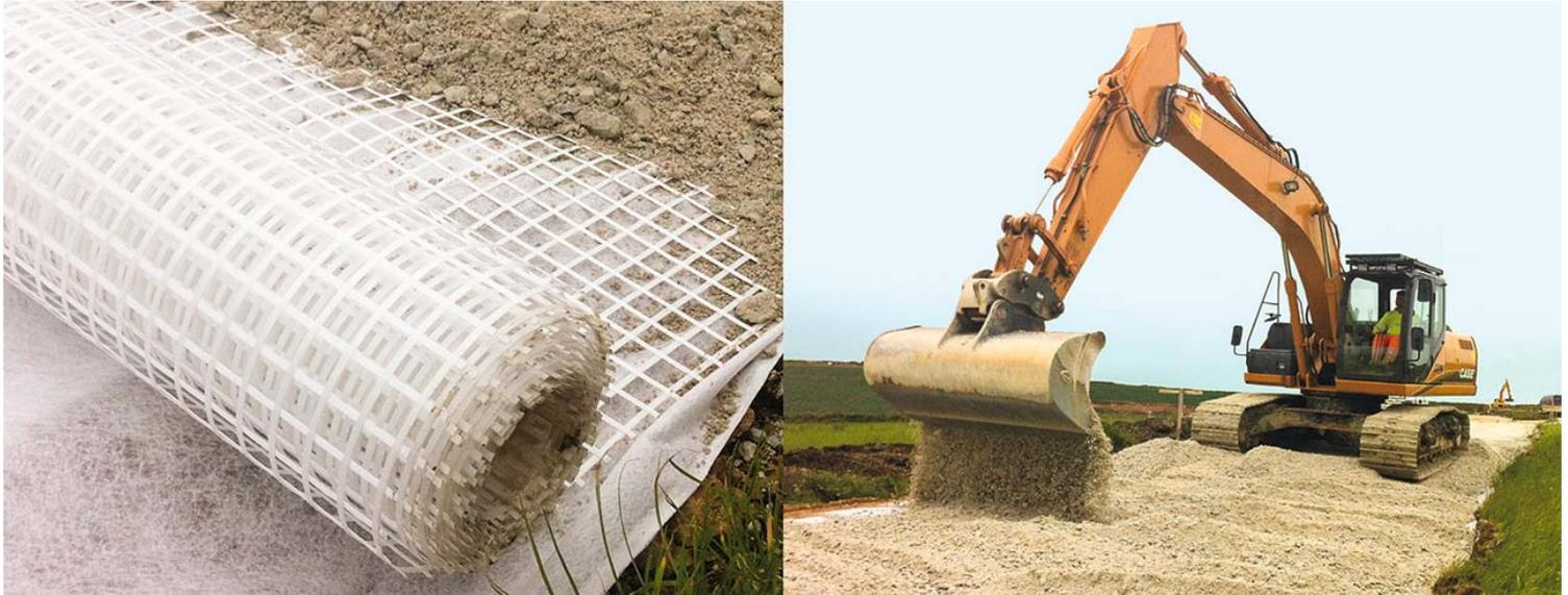
Secugrid® geogrids from Naue proved to be the most cost-effective and technically beneficial solution for the mechanical reinforcement of unbound access roads and crane pads.
