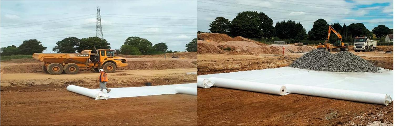
Naue's Combigrig® and Secugrid® products have been used success-fully to significantly improve the bearing capacity of the sub-base prior to construction commencing on site infrastructure for Lancaster University's new £14m Health Innovation Campus.
